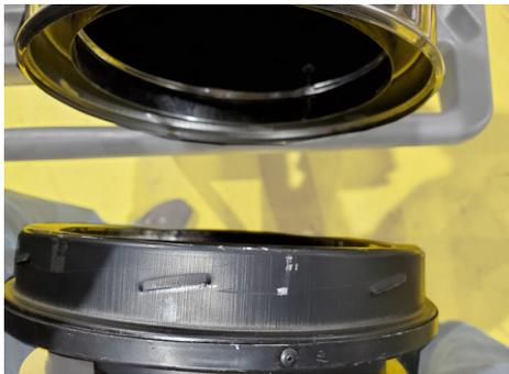
4. Place the chimney cap onto the top of the 8-inch ID chimney section. Twist clockwise until it locks into place. Installation is complete.
